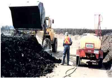
Stock Pile Treatment
